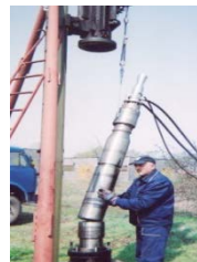
Fig. 12. Driving pilots
